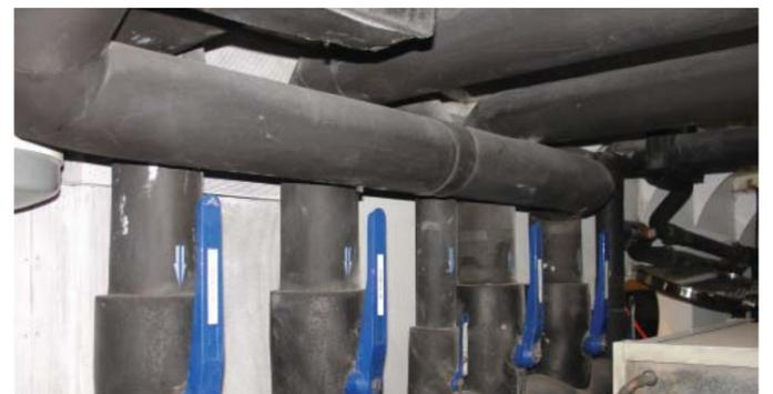
Image 5: This section of duct has insulation missing – as a result condensation and mould growth are forming.
